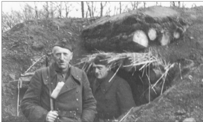
BELOW This Volkssturm platoon leader has properly emplaced his command post bunker on the reverse slope of a ridge to shelter it from enemy fire. (Courtesy of W. Darrin Weaver Collection)
