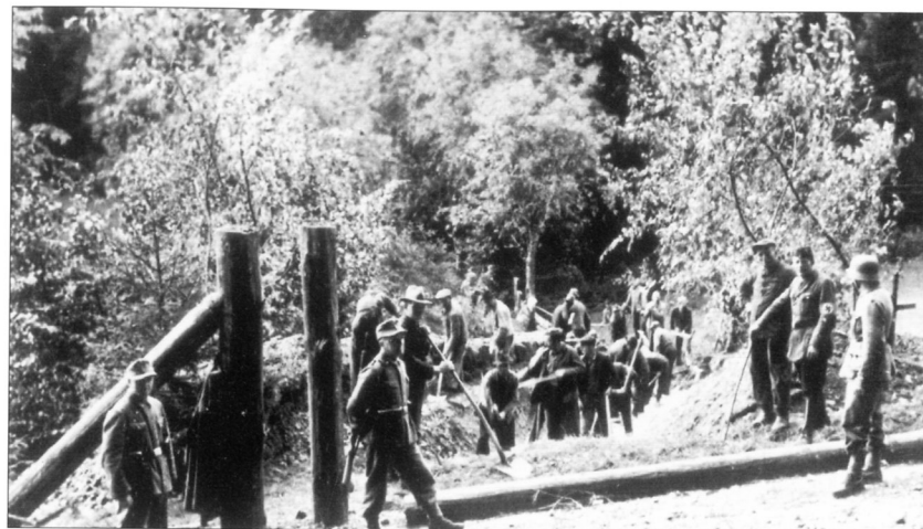
RIGHT Volkssturm men cut and haul tree trunks for a typical rural roadblock. The vertical supports are already in place and additional logs will be inserted horizontally to block the roadway. Army engineers and a Party official supervise. (Courtesy of Bundesarchiv-Bildarchiv Koblenz)
