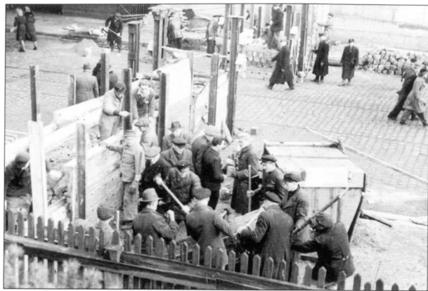
ABOVE Urban Volkssturm men construct a roadblock at a railway overpass in Berlin. These men employ metal beams for the vertical supports, heavy boards as the horizontal walls, and readily available rubble between the walls. Note that the center remains open to traffic. (Courtesy of Bundesarchiv-Bildarchiv Koblenz)
