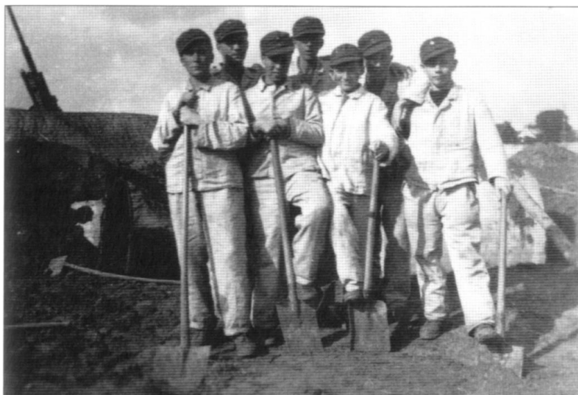
Flakhelfer often spent much of their time on labour tasks, repairing or maintaining their installations. This group, photographed in September 1943, seems to be building a concrete-lined shelter. They wear Luftwaffe fatigue uniforms with their Luftwaffenhelfer caps. (Author's collection)
