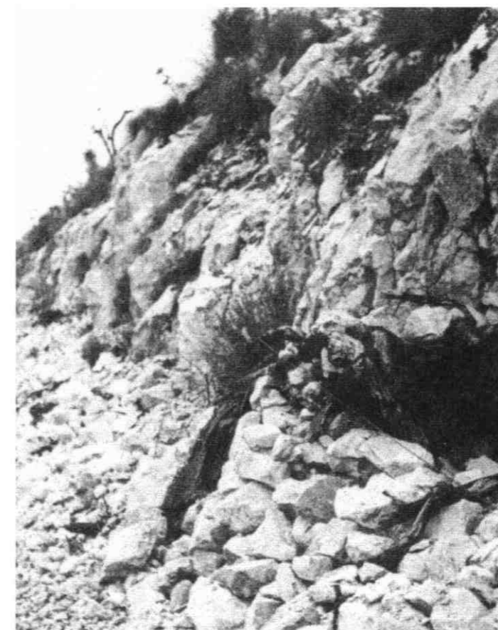
A position built of rocks in the Cassino area.
