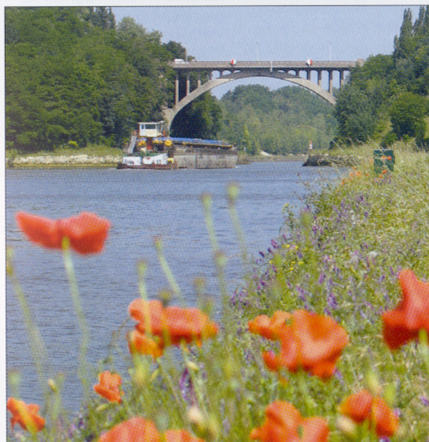
The significance of the high bridge over the Albert Canal at Vroenhoven can be appreciated from these photographs. If it had been demolished, along with the similar high bridge at Veldwezelt, it would have taken considerable time and engineer effort for the Germans to replace them with approach roads down to the canal sides and pontoon bridges across it.
