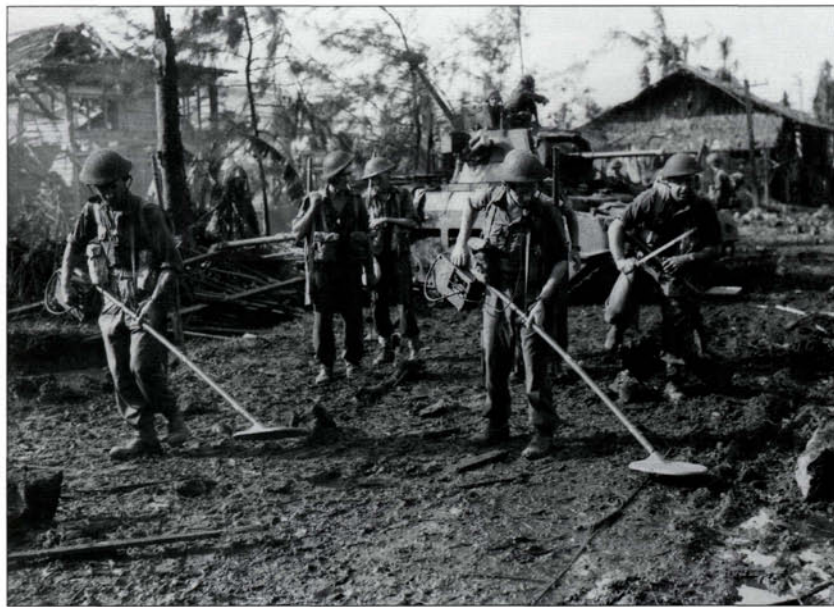
Balikpapan, 1 July 1945: Australian sappers clear the way for a Matilda. Two have mine detectors, while a third is about to prod with a bayonet. Engineers made safe nearly 8,000 mines, booby-traps and unexploded bombs at Balikpapan. By 1945, sappers comprised 9 per cent of the Australian Army – nearly twice the figure in 1941. This expansion took place to meet the demands of campaigning in undeveloped areas, and of providing base services that in the Middle East had been handled by the British. (Australian War Memorial 110379)
