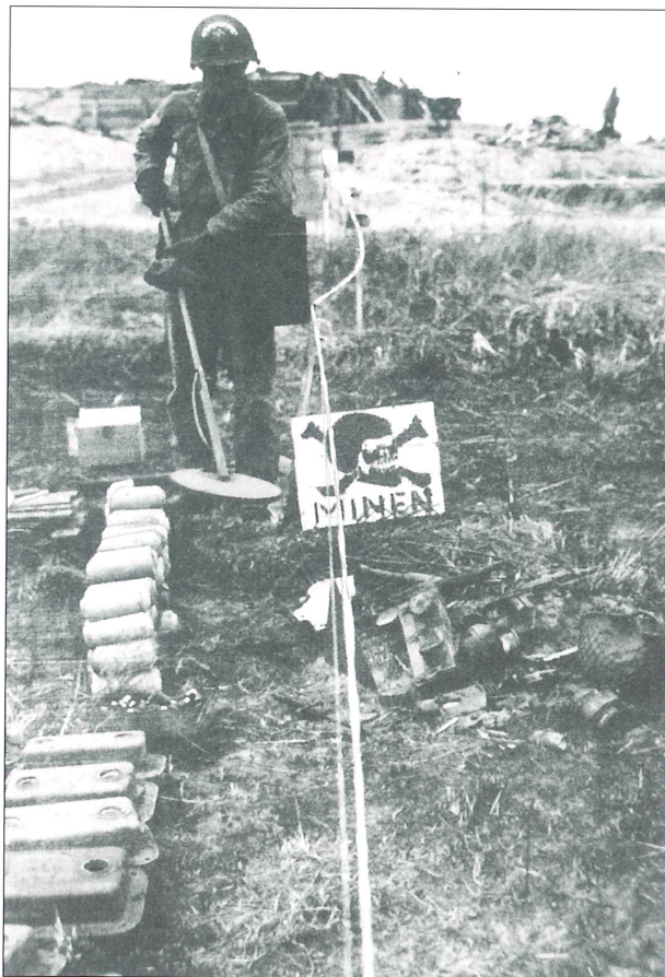
Both beach and shore parties cleared obstacles and mines. Here a soldier of an Army Engineer Special Brigade – identified by the arc painted on his helmet – readies an SCR-625 mine detector before entering a minefield marked with a black-on-white German warning sign. Numerous former French mines have already been lifted and stacked, left.
