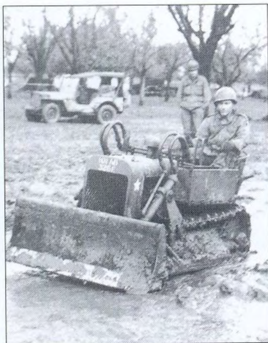
This diminutive bulldozer could be loaded in a transport or heavy glider, but it offered engineers only the barest of earthmoving capabilities for repairing captured airfields. The marking above the grill identifies it as belonging to the 101st Abn Div's 326th Airborne Engineer Battalion.
