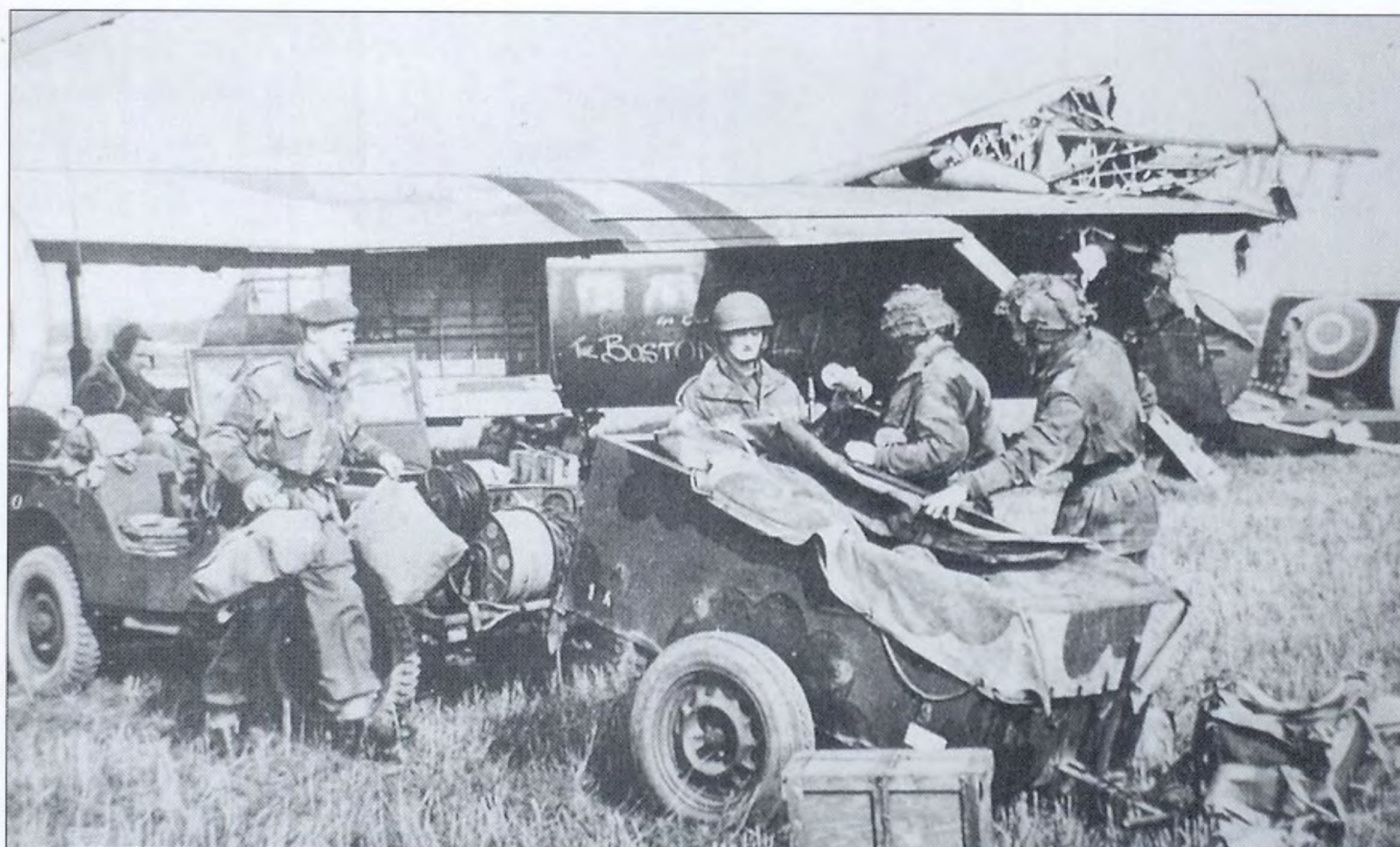
The British Airspeed Horsa glider was designed so that the rear fuselage and tail section could be removed behind the wings for loading and unloading large cargoes. Even when gliders were damaged on landing, equipment could still be salvaged from them. This Horsa, photographed near Arnhem in September 1944, has the tail assembly removed to drive off a jeep and trailer; troops and cargo off-loaded through the drop side door aft of the cockpit (seen here above the jeep windscreen). A Horsa could alternatively carry 25 passengers or an AT gun.
