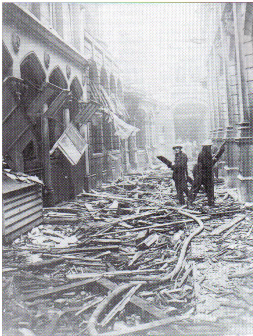
Bomb damage at Austin Friars in the city of London.
