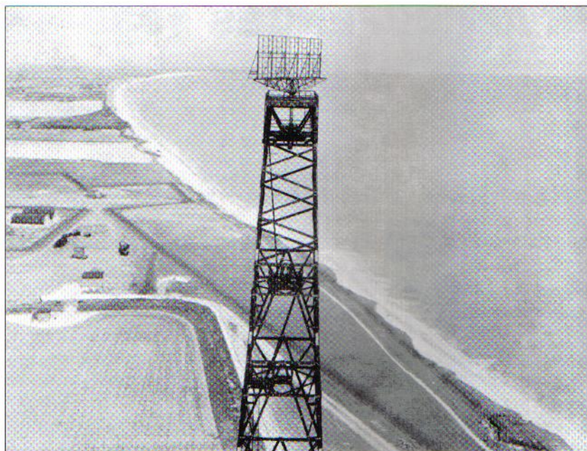
Chain Home Low radar scanner, mounted on top of a 185ft high tower. This radar entered service during the early months of the war, and partially filled the gap in the radar coverage at the lower altitudes. The CHL could detect aircraft flying at 500ft out to 18 miles, and aircraft flying at 2,000ft out to 35 miles.
