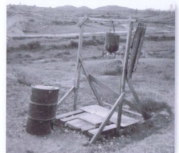
A crude field shower facility. The 3-gallon canvas shower bag was tuned on and off by turning the large shower head, which surprisingly built up more than adequate water pressure. A good shower could be had with just 4-5 gallons. (John Burford collection)
