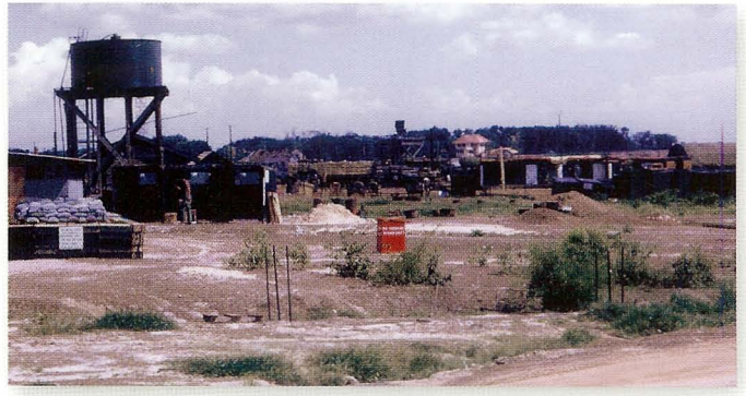
View of a typical larger base for a brigade or division on which many aviation units were stationed. Newly arrived officers would recommend that a machine gun be positioned atop water towers. That only attracted fire, making holes in the tower.
