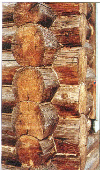
Virtually the same methods of timber construction used in 13th century Russian fortresses are used for some houses in the Russian countryside. This example in Vladimir shows how the tree-trunks were grooved to make a weatherproof fit and to achieve a strong corner. (Author's photograph)
