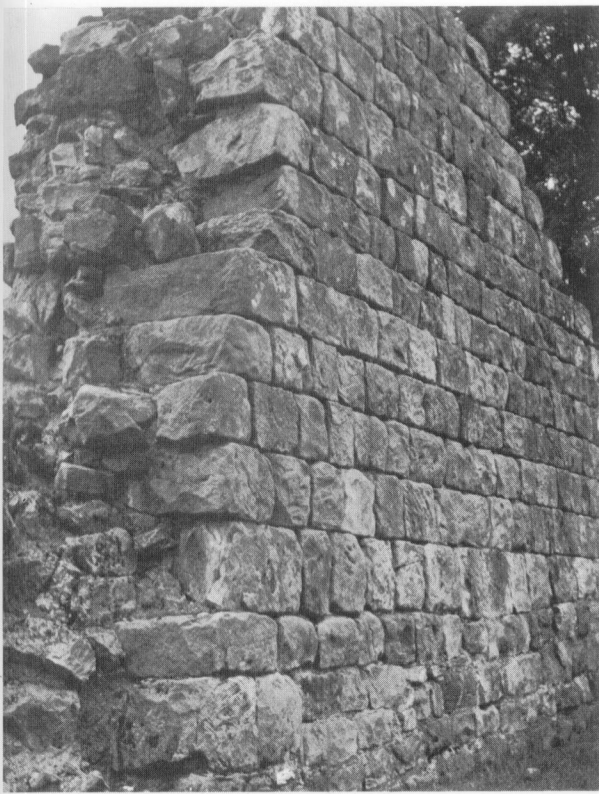
A fragment of the structure of Hadrian's Wall at Hare Hill; the core is original, and the facing stones are restored.
