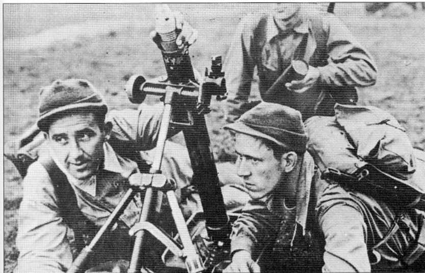
Crew of a US Army 60mm M2 mortar in action on what is obviously a training exercise. Ease of operation and relatively light weight made this a popular weapon with US troops in all theatres of the war. Note the man in the background holding another round of ammunition still in its tin carrying case. (IVH)
