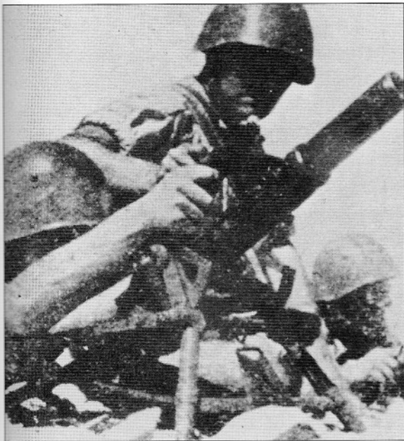
The Italian Army's Brixia Model 35 mortar in the unusual calibre of 45mm. Extremely complicated when compared to other similar weapons, the Model 35 was not highly rated by the Italian troops who had to use it. It is believed to have only seen very limited action in the early part of the Libyan campaign. (IVH)
