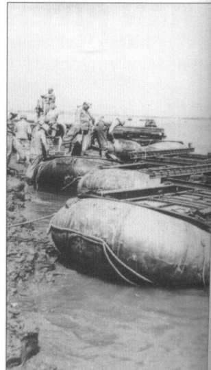
Marines from the 1st Engineer Battalion assemble pontoon rafts into two 50-ton-capacity rafts to ferry tanks and vehicles across the Han River. Insufficient pontoons were available to span the 400yd-wide river. (USMC)
