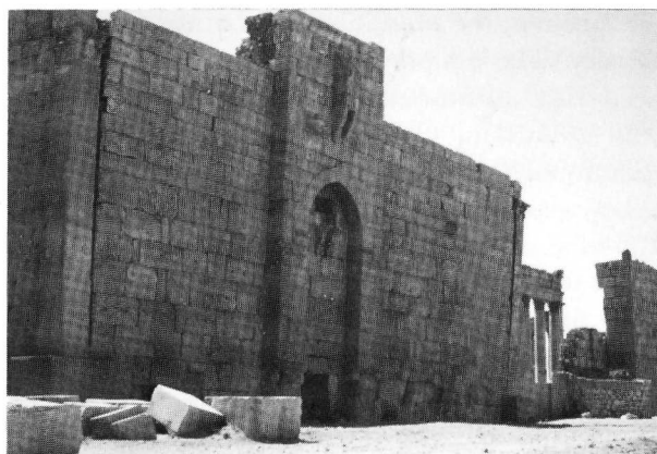
In AD 1132 the huge Temple of Bel in Tudmir was turned into a fortress to defend this strategically vital oasis. Its main door is protected by a simple machicolation.
