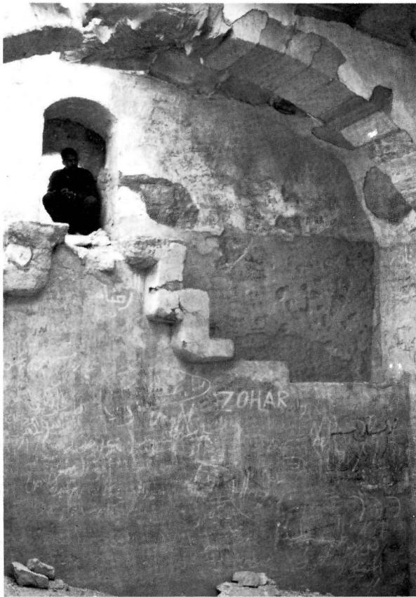
Saladin's great mountain-top castle of Qalaat al Jindi overlooks the main pilgrim route across Sinai. This shows one of at least three underground water storage cisterns, vital in such a desert area.
