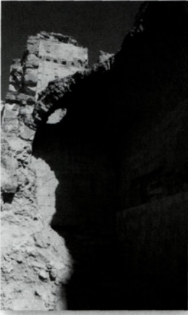
The chamber that ran inside the main wall around the smaller fortified enclosure at Qasr al-Hayr al-Sharqi incorporates both stone and brickwork, the masonry being used for the walls whereas the vaulted roof is of brick. (Author's photograph)
