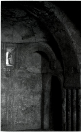
Qasr al-Kharana includes several features deriving from Iraqi, Iranian and Central Asian architecture, including stucco surfacing, simple arched squinches and rows of decorative false columns supporting the main arch. (Author's photograph)
