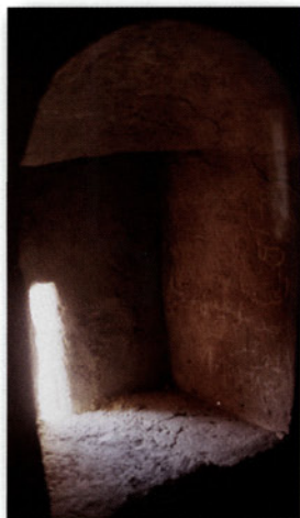
The windows of the early 8th-century Umayyad desert fort of Qasr al-Kharana in Jordan cannot have served as arrow slits. Even where they can be reached from inside the building, as here, the 'arc of fire' is too narrow to be militarily useful. (Author's photograph)
