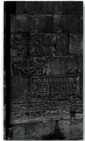
Some medieval Islamic fortifications in the Middle East were decorated with carved animals and other motifs as well as Arabic inscriptions. Those seen here are on the 'Dark Gate' of Diyarbakr, which was substantially rebuilt during the 11th century. (Author's photograph)
