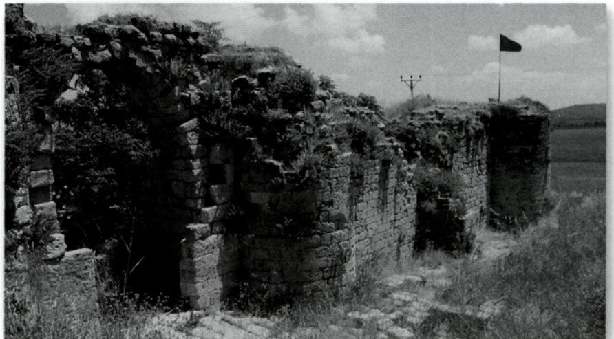
By the 9th or 10th century, when the surviving walls, towers and entrance gate of Kfar Lam were renovated, the old Romano-Byzantine tradition of mixed brick and stone had largely been abandoned by the Muslim military architects of Syria. (Author's photograph)
