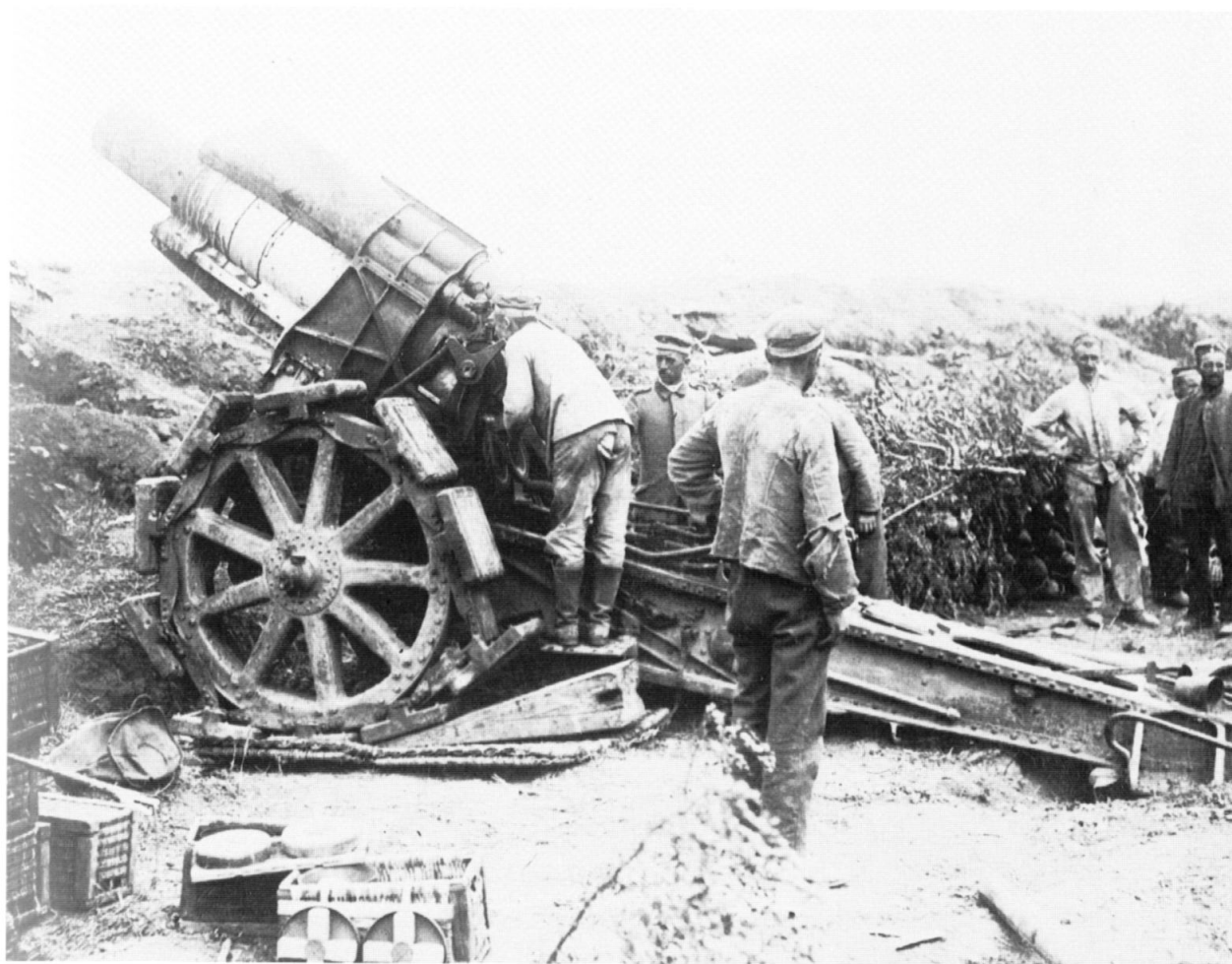
A German 21 cm howitzer with slats on its wheels to reduce the recoil. Even with the spade trailer dug in and wedges under the
