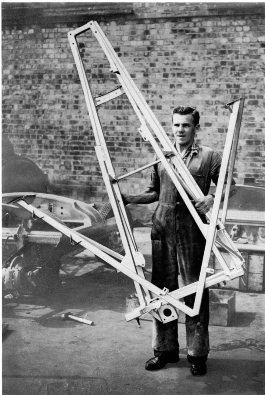
25 The tubular front sub-frame of the sports/racing Jaguar D-type, used in conjunction with a stressed skin body. A similar type of construction is found in the road-going E-type Jaguar
