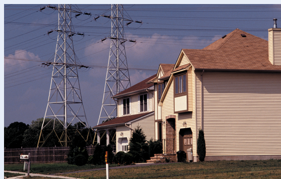
High-voltage power lines such as these emit low levels of 60 Hz electromagnetic radiation (also called ultralow frequency , or ULF, radiation). (Martin Heitner/Stock Connection Worldwide/NewsCom.)
